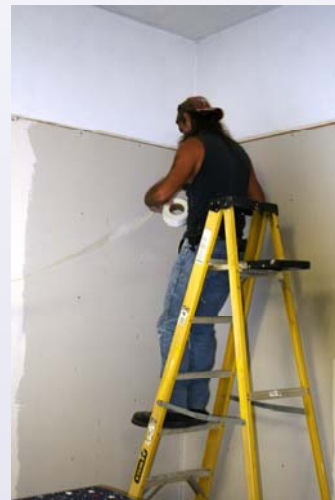
Tim Ayers taping the drywall (left) and Barry Costner sealing the joints (right). Tim Ayers caulking the joints (below).
