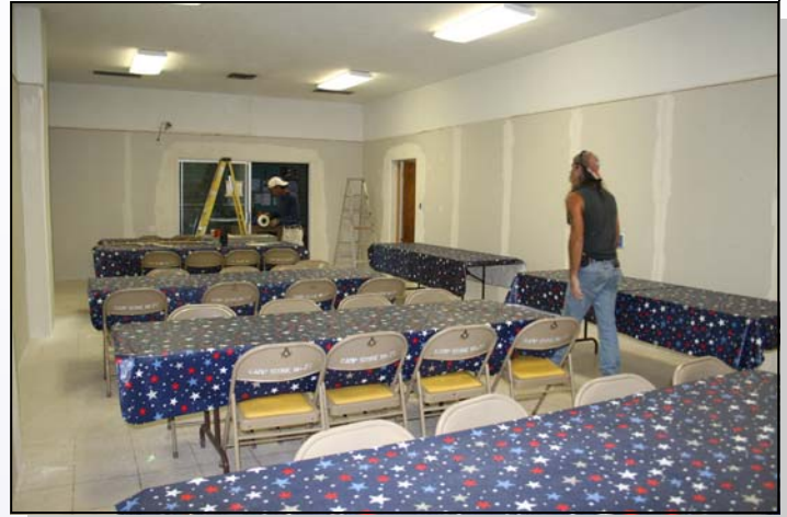
Barry Costner and Tim Ayers inspect the drywall
