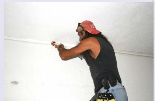
Tim Ayers taping the drywall (left) and Barry Costner sealing the joints (right). Tim Ayers caulking the joints (below).
