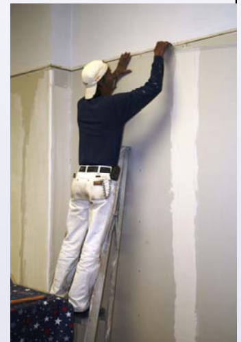
Tim Ayers taping the drywall (left) and Barry Costner sealing the joints (right). Tim Ayers caulking the joints (below).
